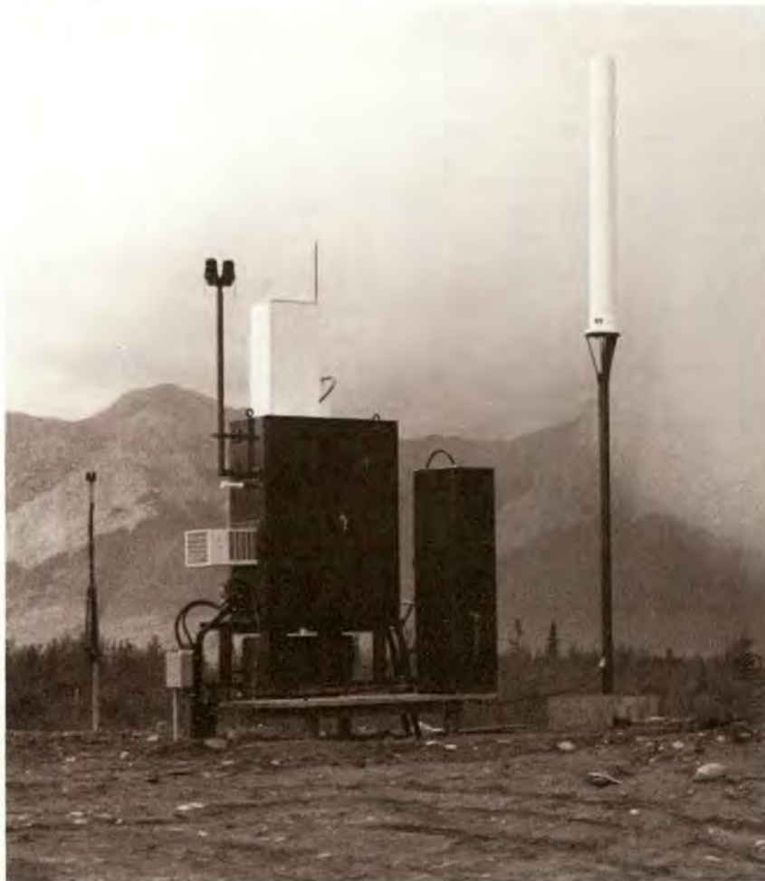
The MLS is a very compact precision approach system that requires very little site preparation. The only requirements are a concrete pad and proper electrical power. This elevation station is at Jasper-Hinton, Alberta, Canada. Photo courtesy of Hazeltine Corporation.
