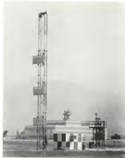
Compare this ILS glide slope antenna and equipment shelter with the MLS elevation antenna on the previous page. The MLS is more compact, more reliable, and more versatile.
